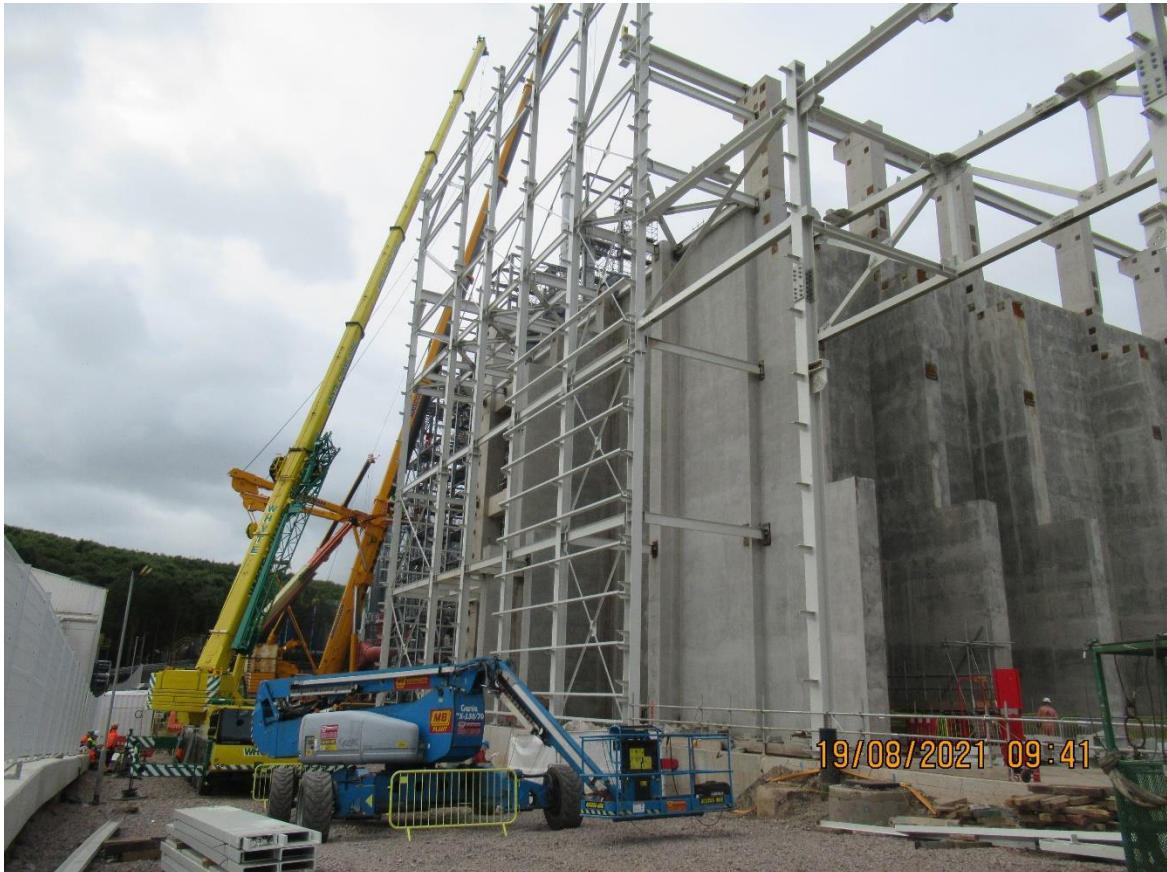
Waste Bunker and Building Steel Structure
