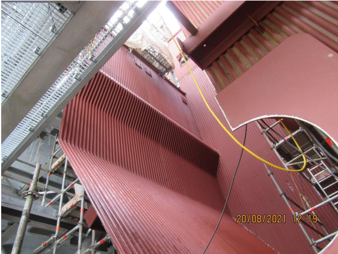
Boiler Construction Underway
