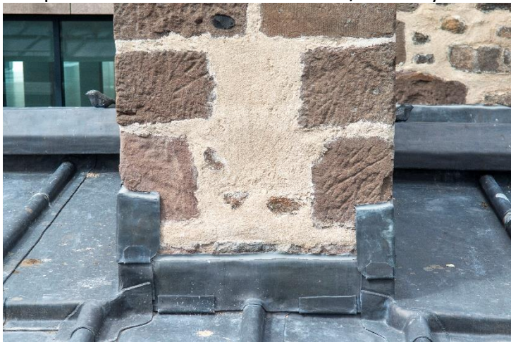
Leadwork detail of roof
