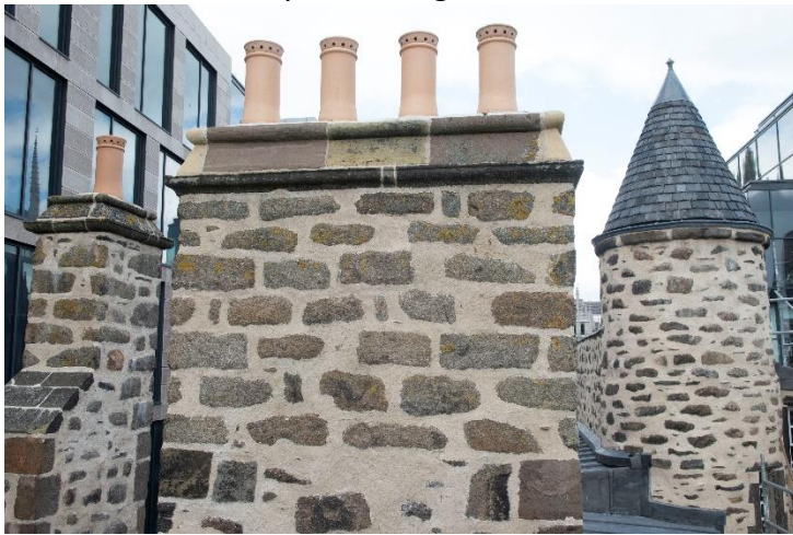
Completed refurbishment of the roof / chimneys
